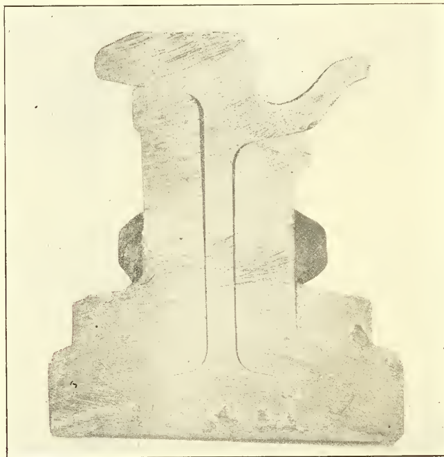
FIG. 69.—Section through Modified Clark Joint. It will be Noticed that the Lower Part of the Rail and Fish Plates are entirely Amalgamated.
